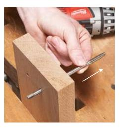
4 Switch to a drill bit that's the root diameter of your tap. Center the bit on the dimple and drill all the way through the wood.
